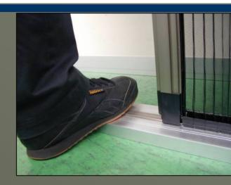
The patented mesh floor guide disappears into the sash mullion when operated leaving a virtually un impeded pathway through the opening.
