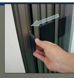
The pleated insect screen mesh incorporates a mid span tensioning cord, that operates the screen and assist keeping the mesh in place during windy conditions
